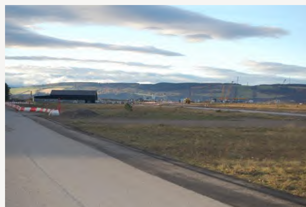
Image 2, 3 and 4: Images showing current construction taking place on the site
