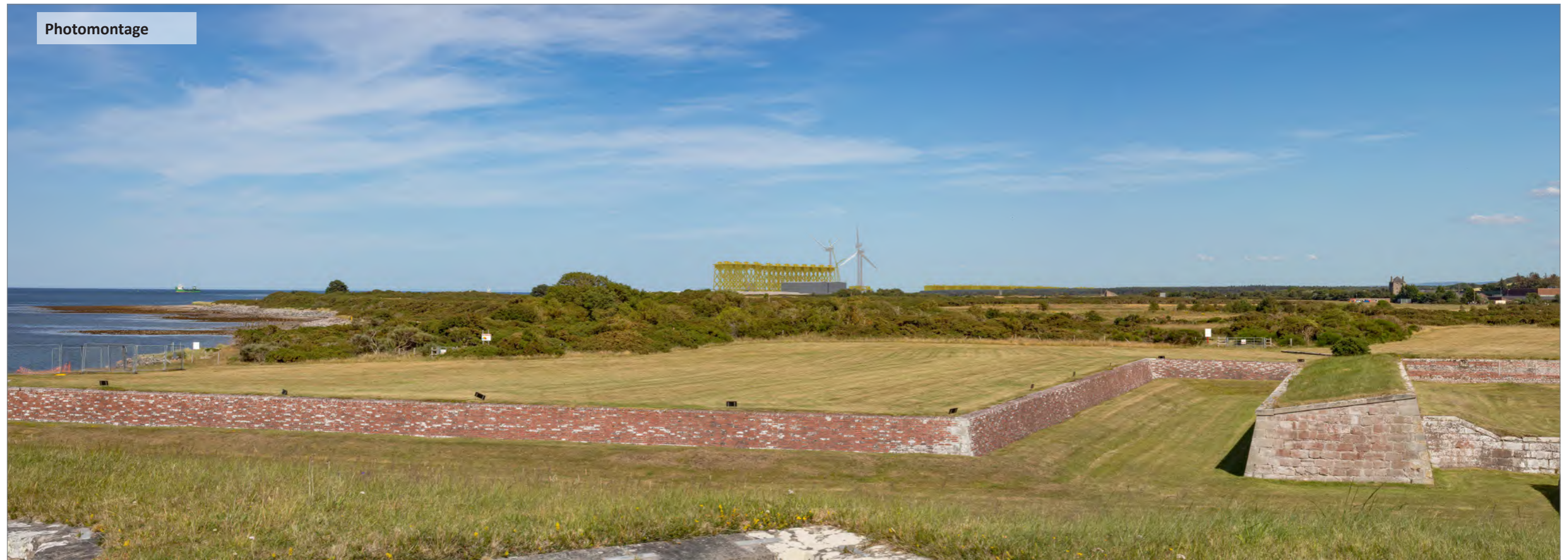
Figure 7.5.4b - Viewpoint 04 - Fort George - north east bastion
