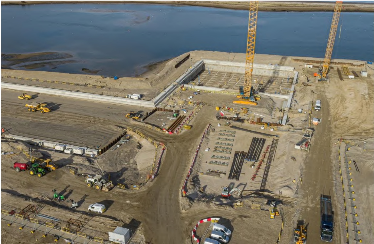
Image 3.1: View of Consented Port during Construction
