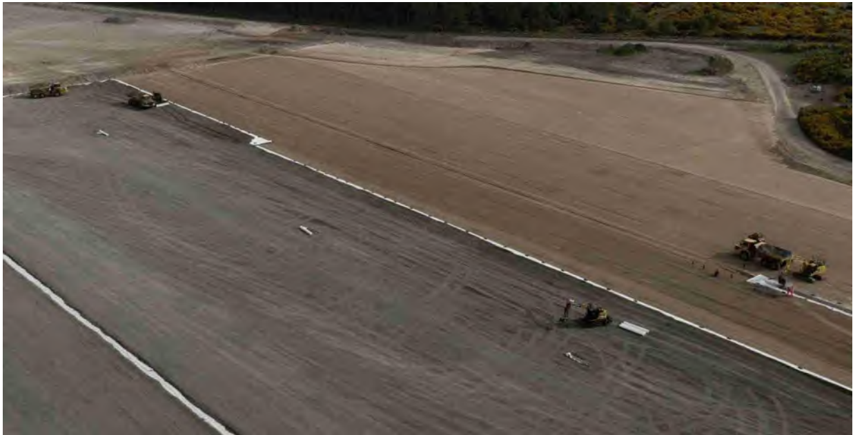
Image 3.3 Land Raising and Creation of Working Platform
