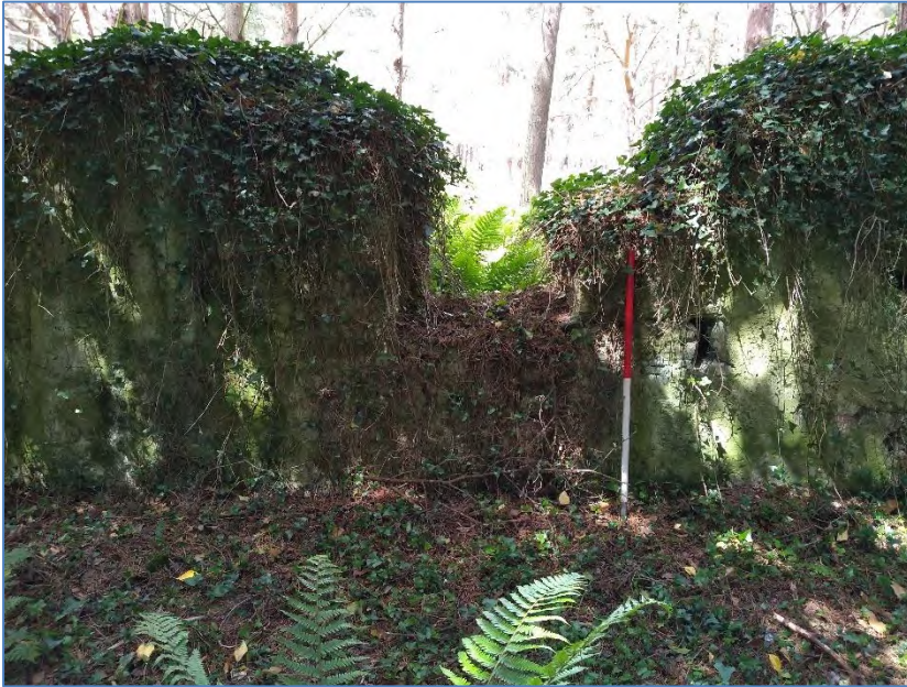
Image 8: ORCA 09, north wall of the building with window, looking north
