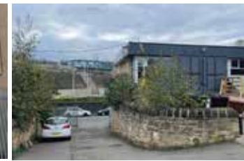
Rear of the vacant social club building from within the site
