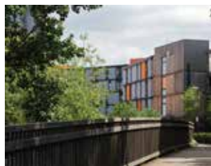
Westfield Avenue Housing, Edinburgh 7N Architects
