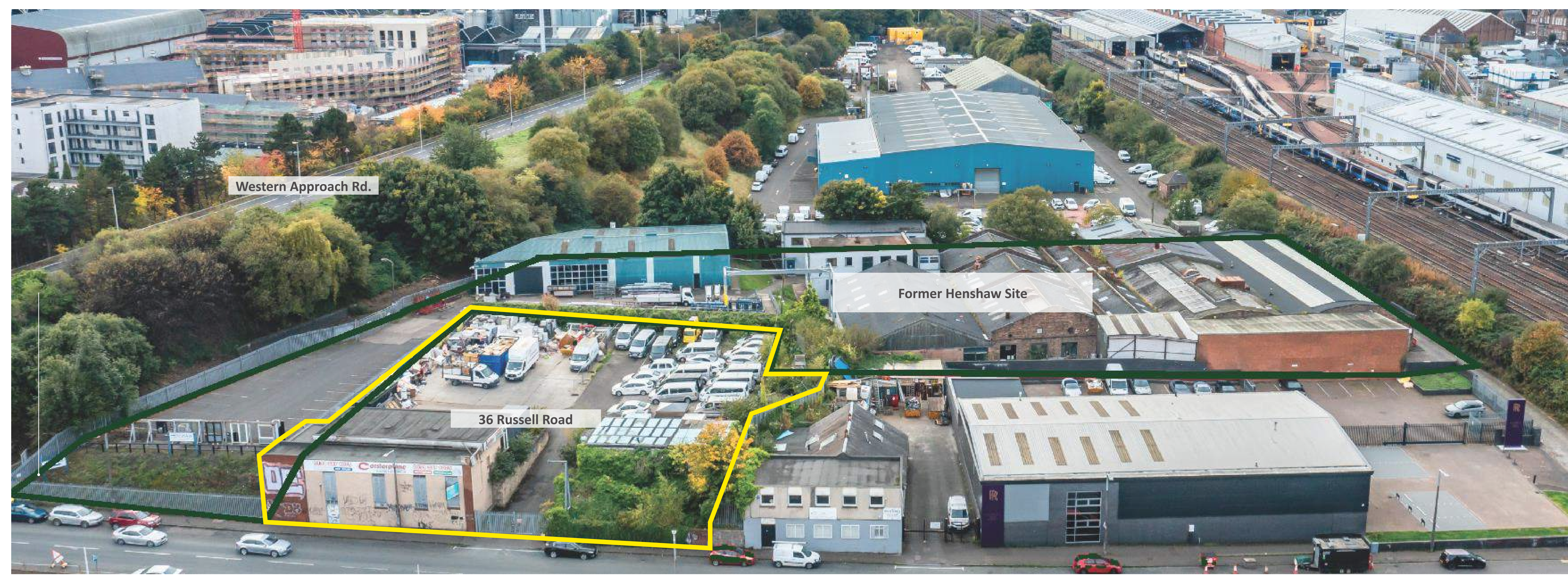
The Existing Site - Aerial looking West
