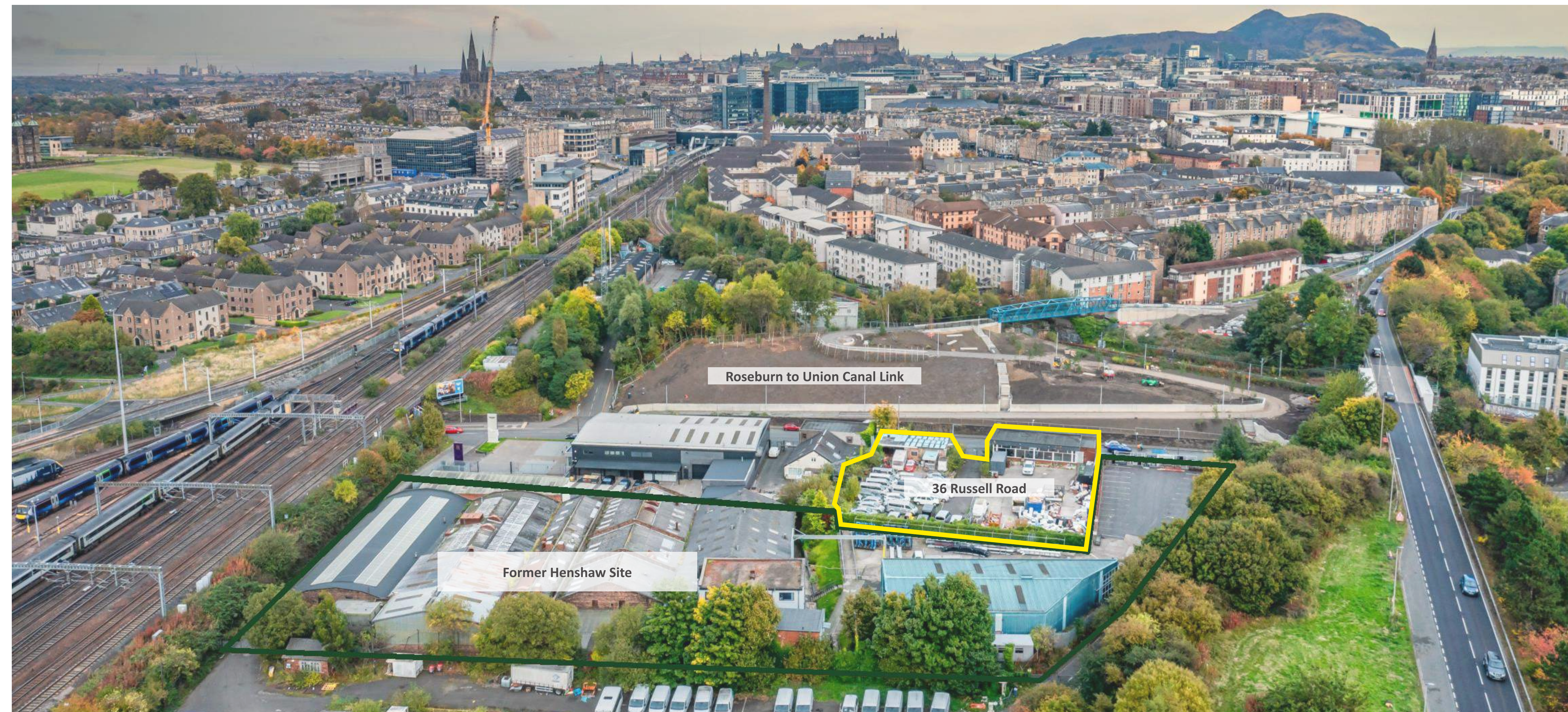
The Existing Site - Aerial looking East
