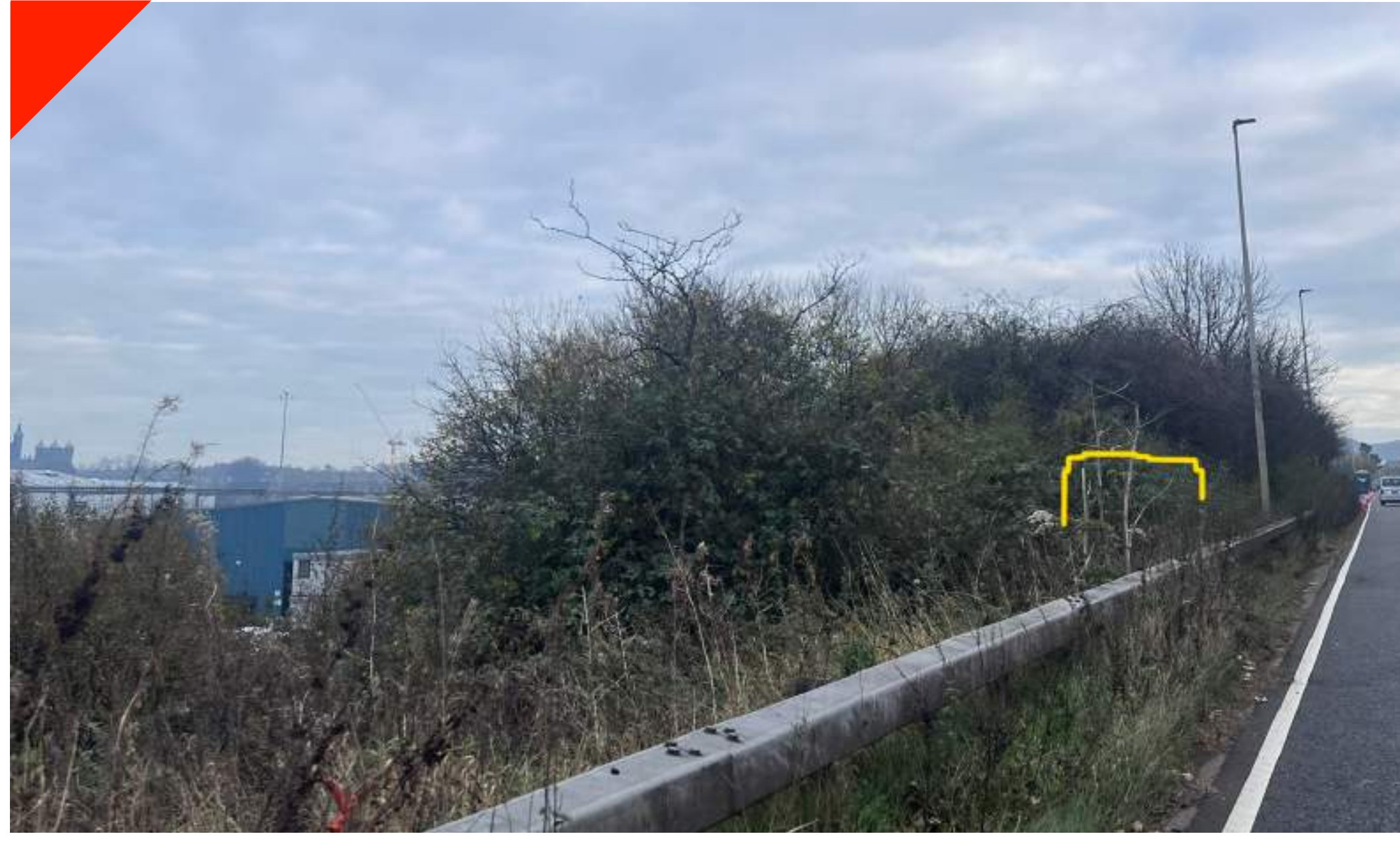
3 - Long Distance View - West Approach Road looking East
